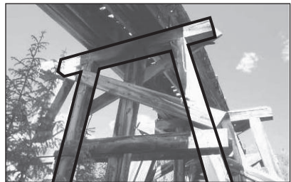
Above: The bent on a trestle bridge is key to giving the structure its integrity.
