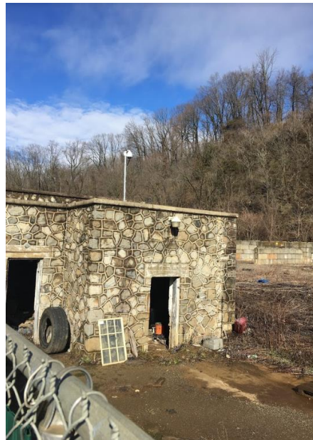
Photograph 18. East face of Building 3 above fence, Photo Taken April 1, 2017.
