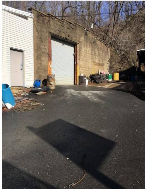
Photograph 2. East Side of Building 1, Photo Taken April 1, 2017.
