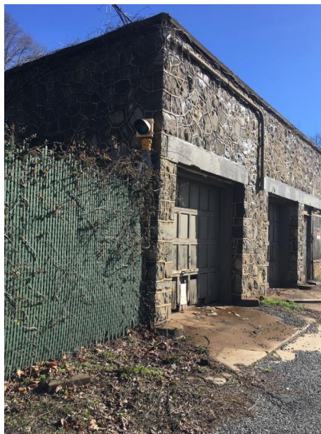
Photograph 16. Front of Building 3, Photo Taken April 1, 2017.
