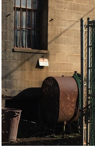
Photograph 5. South Side of Building 2 showing oil tank, Photo Taken April 1, 2017.
