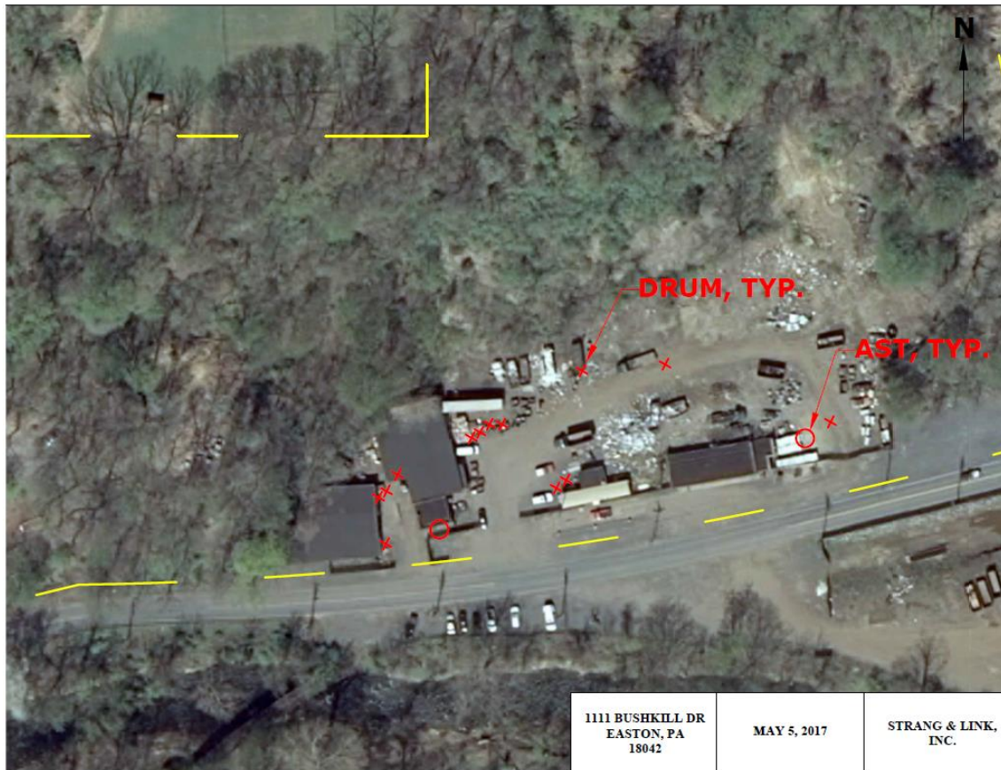
Figure 110: Location of Drums and ASTs on Subject Property
