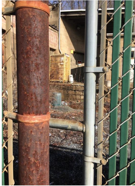
Photograph 7. East Side of Building 2 through fence, with unidentified substance container, Photo Taken April 1, 2017. Easton Iron & Metal Phase I Environmental Site Assessment, May 8, 2017.
