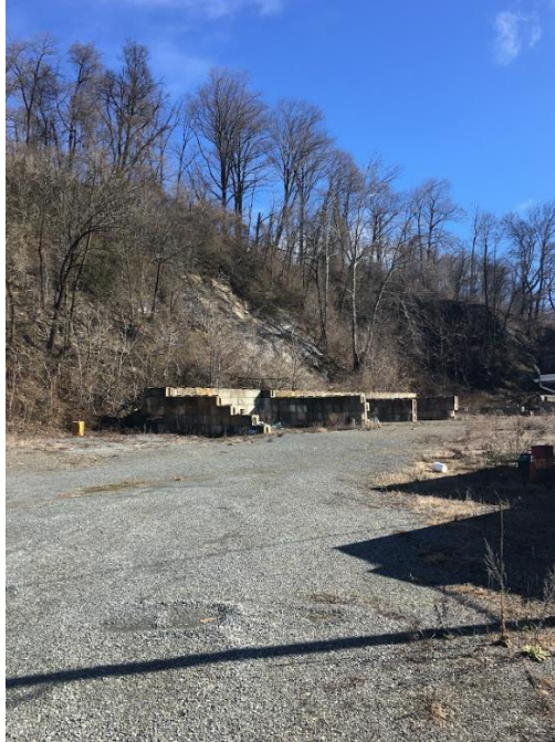
Photograph 13. Bays in center of property above fence, Photo Taken April 1, 2017.
