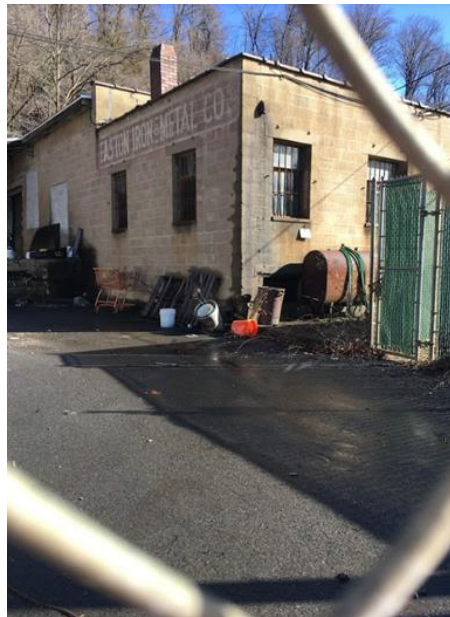
Photograph 4. West Side of Building 2 with oil tank, Photo Taken April 1, 2017.
