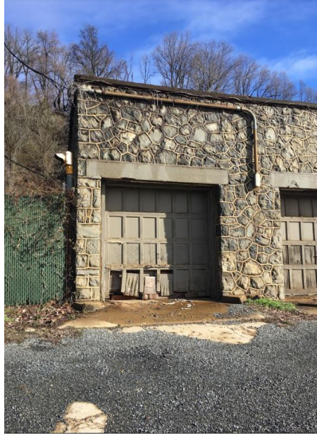
Photograph 17. Front of Building 3, Photo Taken April 1, 2017.
