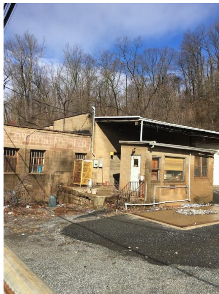
Photograph 6. East Side of Building 2, Photo Taken April 1, 2017.
