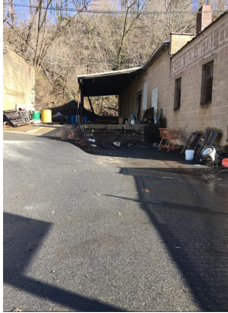
Photograph 3. West Side of Building 2, Photo Taken April 1, 2017.
