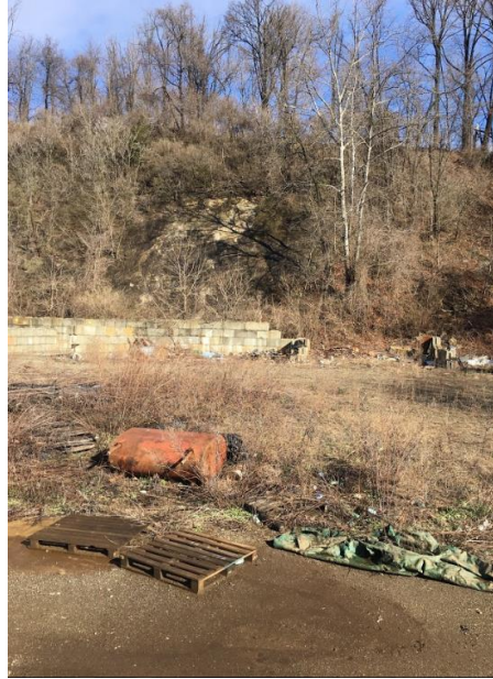
Photograph 19. Deserted aboveground storage tank above fence, Photo Taken April 1, 2017.
