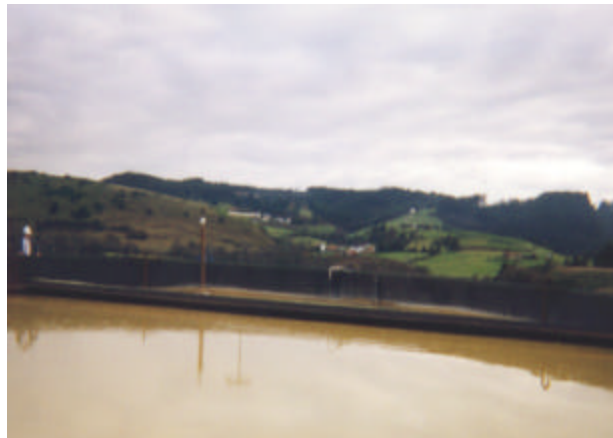
Sanitaire's SBR wastewater treatment system is used to clean a very complex waste stream at a Dupont Corporation chemical facility in Northern Spain.
