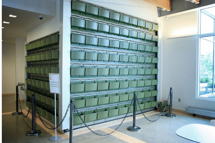
Figure 24: LiveWall Infrastructure (LiveWall, LLC “How to Install a Living Wall from LiveWall,” n.d.)
