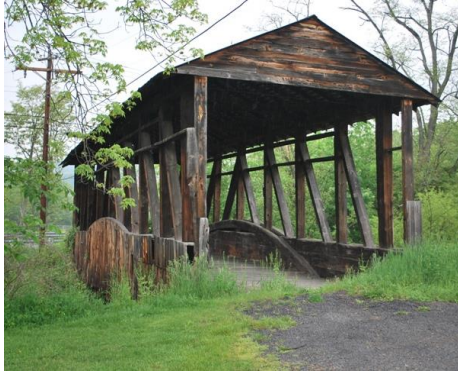
Figure 19: Space covered by complete roof (“Covered Bridges of Pennsylvania”, n.d.)
