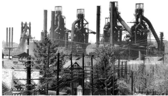
Figure 5: Bethlehem Steel Company (Radzievich, 2018)
