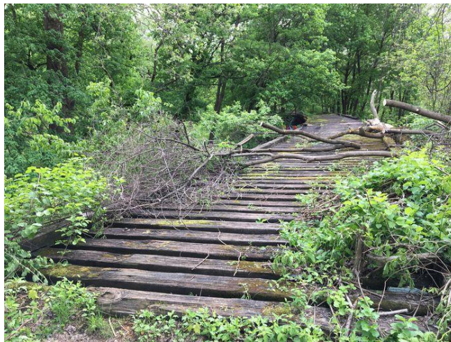
Figure 3: Current state of the bridge (Bresswein, 2019)
