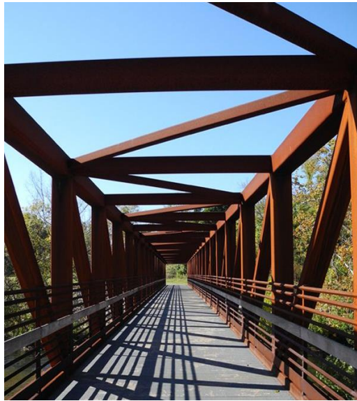
Figure 18: Partial Roof (“Wasena Park pedestrian bridge over the Roanoke River”, n.d.)
