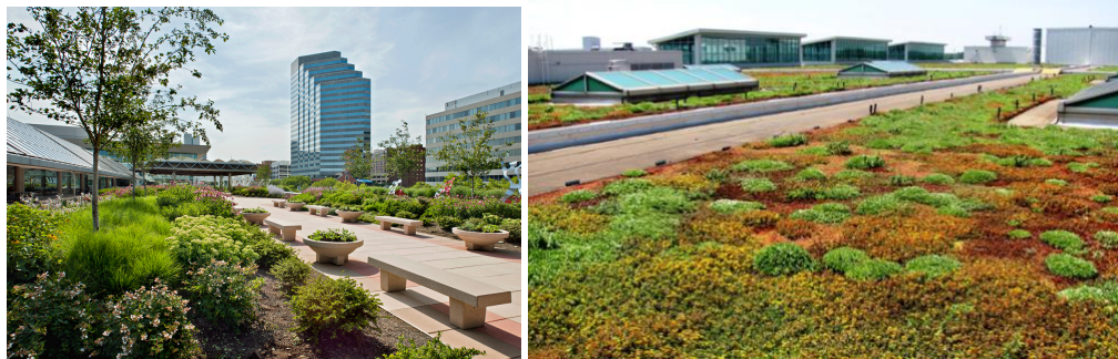
Figure 18. An Example of an Intensive Green Roof with Specific Areas for Community Members to Gather. Adapted from Baltimore Convention Center , Greenroofs.com, 2018
