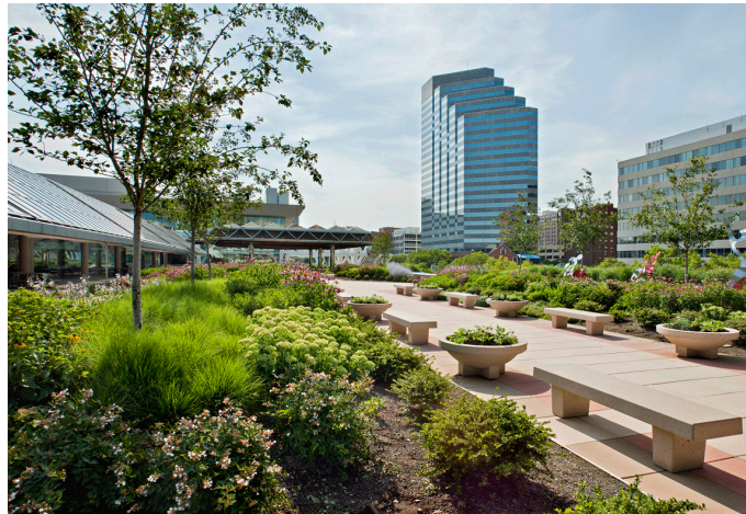
Figure 1. An Intensive Green Roof with Areas for Community Members to Gather. Adapted from Baltimore Convention Center, Greenroofs.com, 2018.
