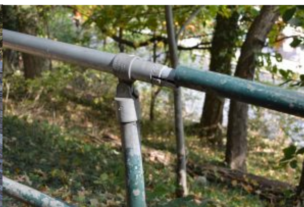
Figure 7: Current State of Railing
