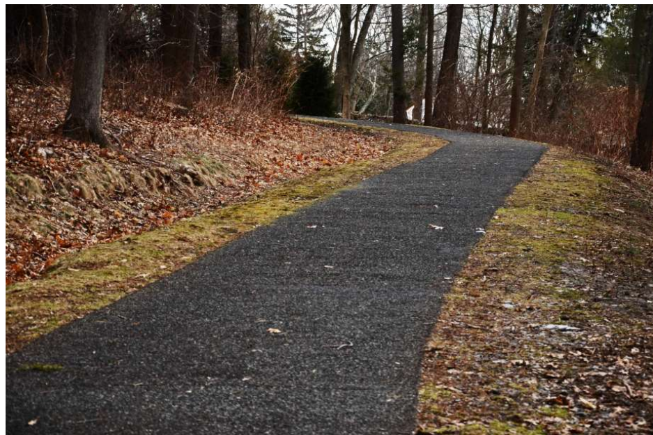
Figure 5: Flexi-Pave, to be used for ramps.
