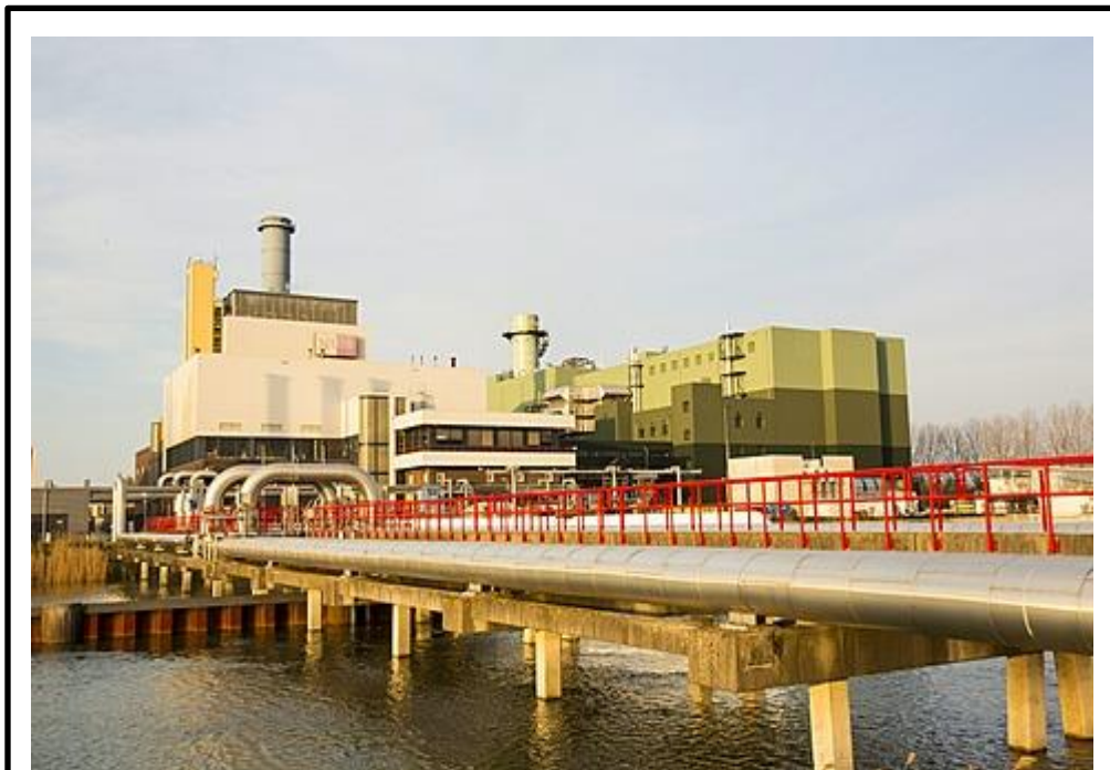
Figure 10: The Diemen CHP plant in Amsterdam, Netherlands. ( https://images.robertharding.com/preview/RM/RH/HORIZONTAL/911-9796.jpg )
