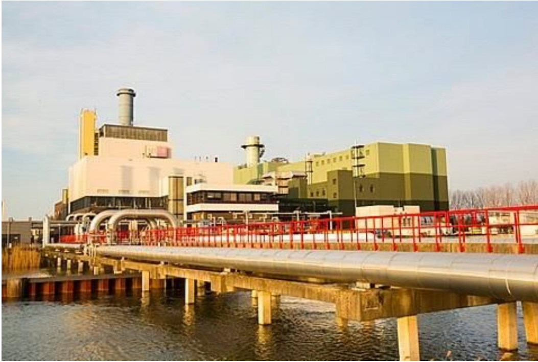
Figure 4: A CHP Plant in the Netherlands; www.robertharding.com
