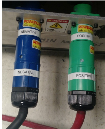
Figure 14. Power Supply Connections
