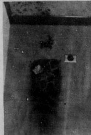
Evidence of arsonist's work in Watson Hall.
