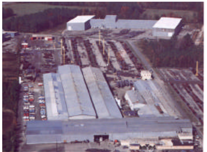
SOUTH CAROLINA P.O. Box 100520, Florence, South Carolina 29501 (843) 662-0381 Joists & Deck Fax: (843) 662-3132
