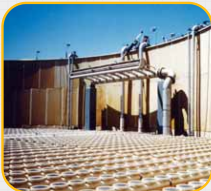
Industrial wastewater treatment plant in circular tanks
