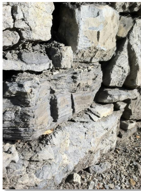
Figure C4. Image of rocks forming the foundation of the retaining wall along College Avenue and Bushkill Drive.
