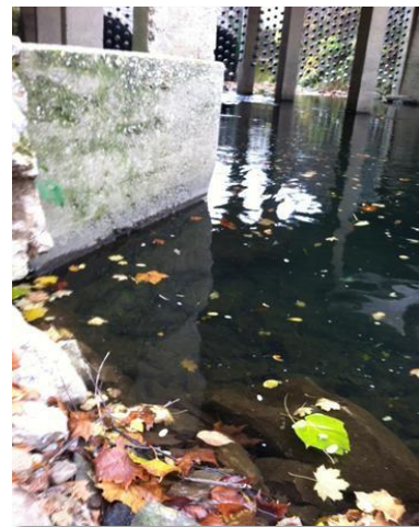
Figure C11. Scour formation under Bushkill Creek retaining wall. Photo taken November 7 th .
