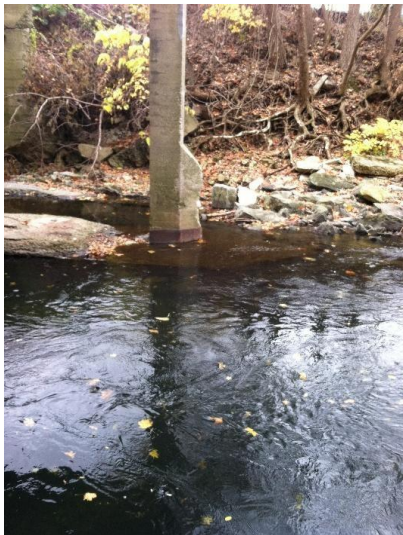
Figure C10. Scour formation under 3 rd St. Photo taken November 7 th .
