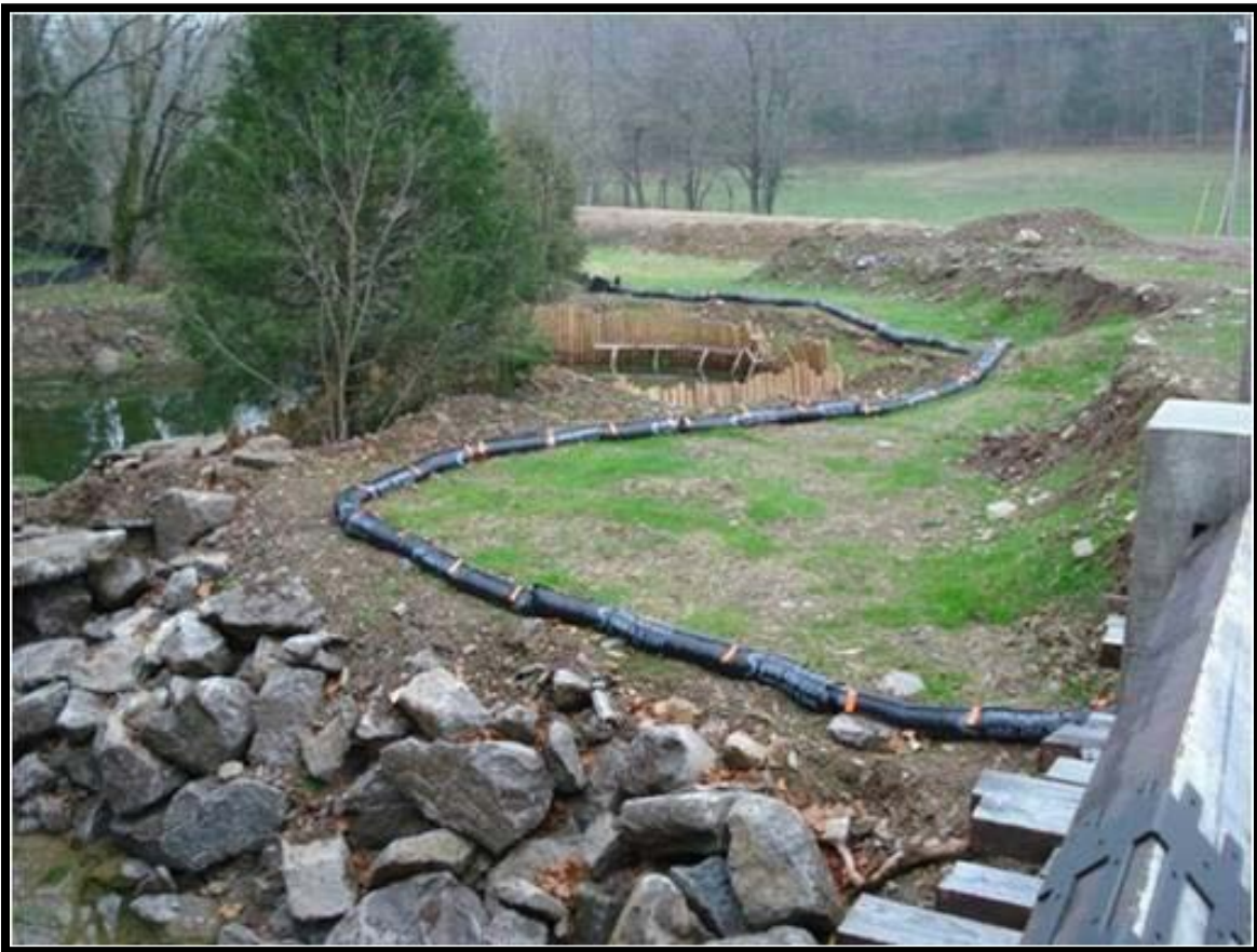
Figure IV.8 Weighted Sediment Filter Tube
