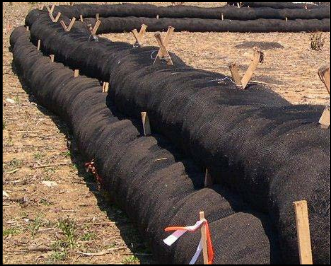
Figure IV.3 Compost Sock Sediment Trap
