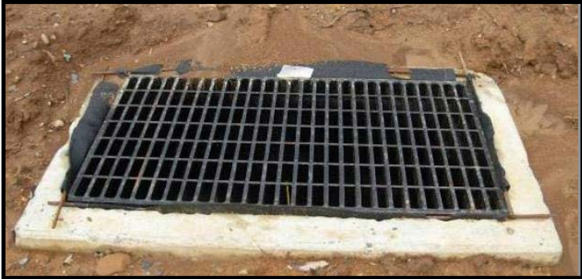
Figure IV.10 Inlet Filter Bag
