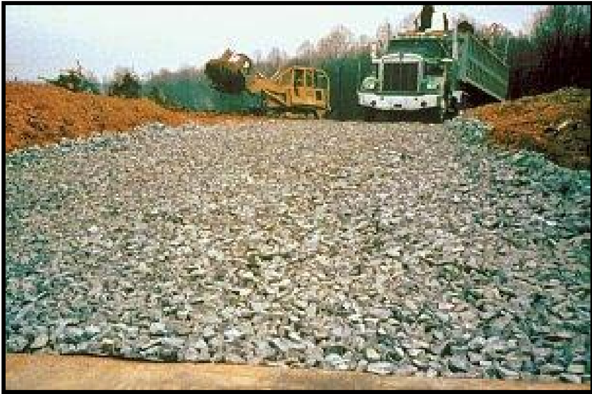
Figure IV.1 Rock Construction Entrance
