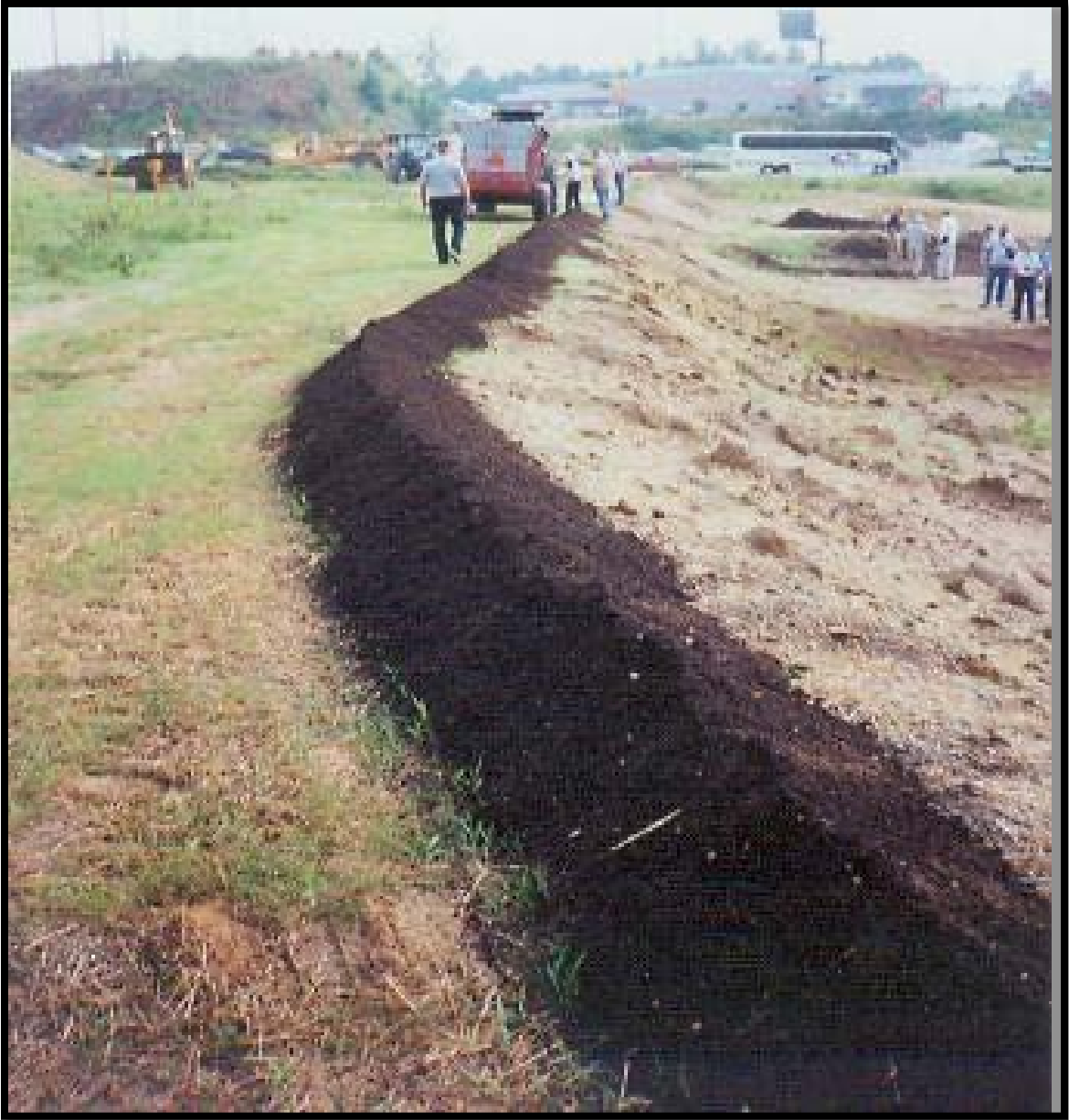
Figure IV.7 Compost Filter Berm
