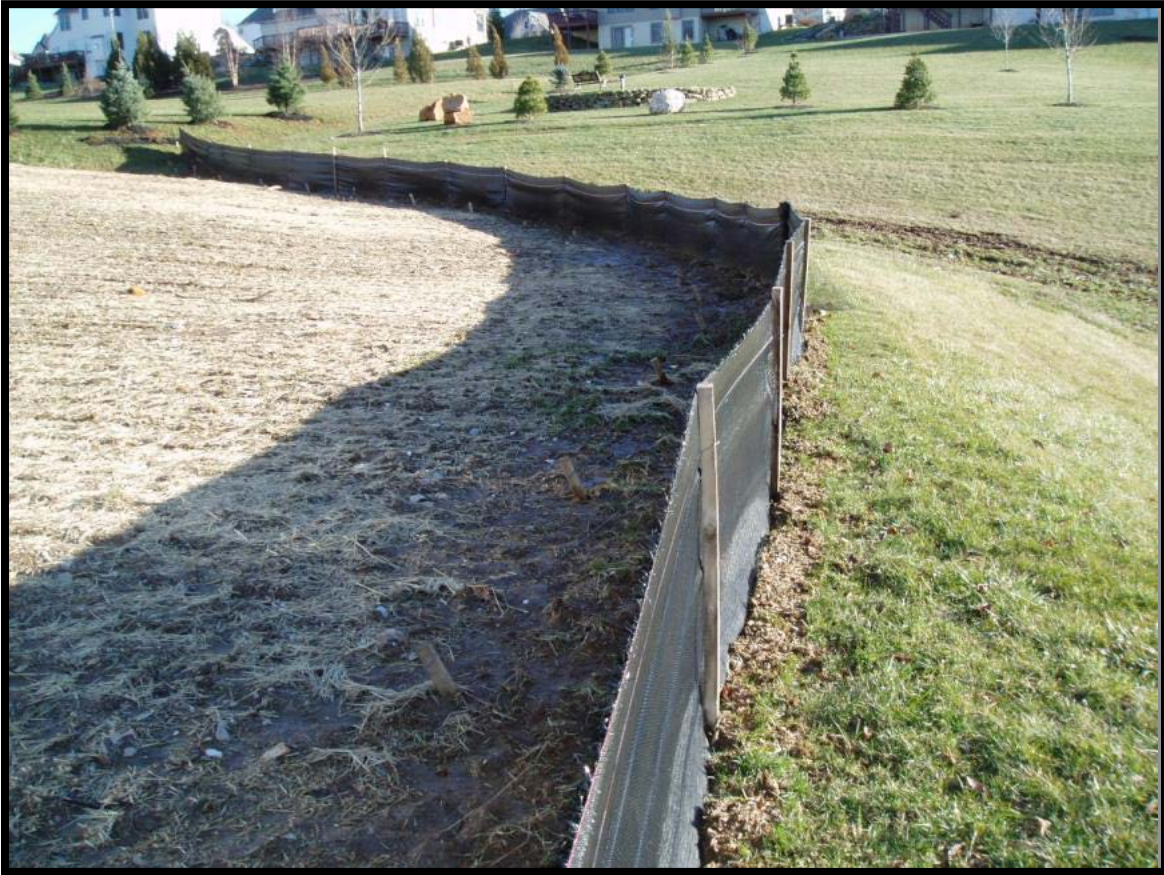
Figure IV.9 Silt Fence
