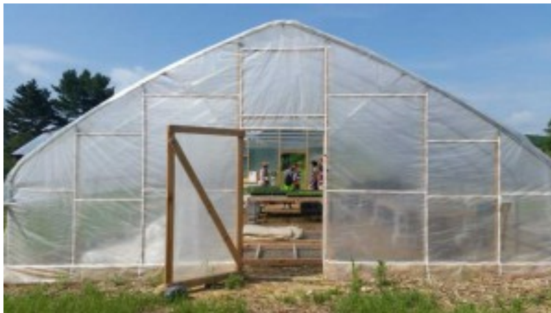
Gothic Framed Passive Ventilation Greenhouse (size of our hoophouse design)
