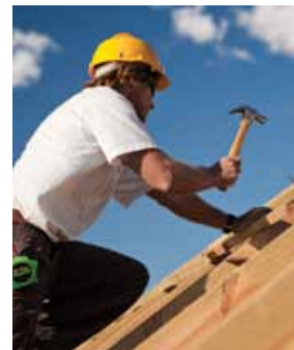
After the storm, repairs were made on 59 homes throughout the Lehigh Valley.
