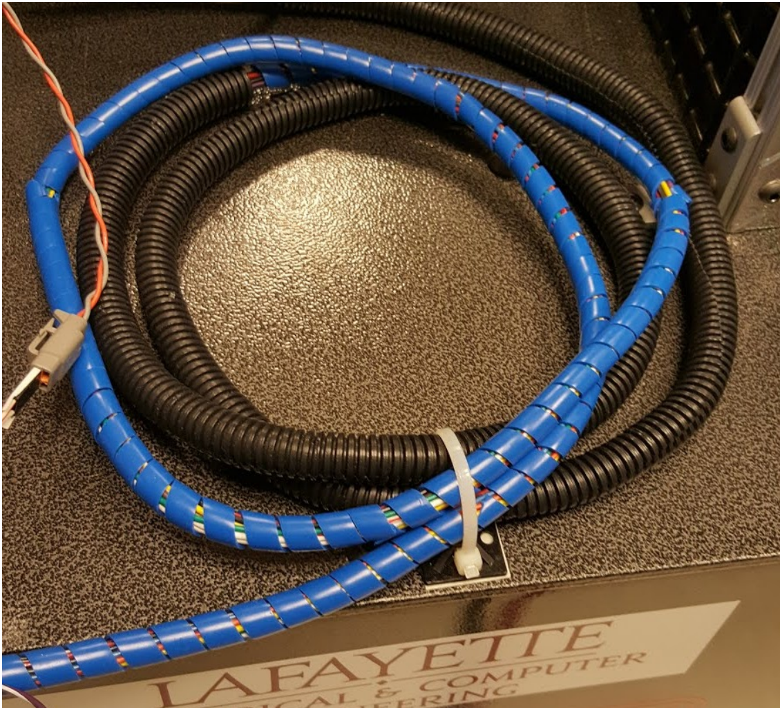
Mechanical securing of motor controller wiring harness.
